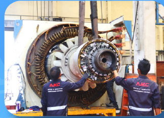
Repair Rotor Generator " ABB " 45,800 kVA. 2,299 A. 1,500 RPM.
