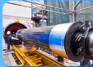
Rewinding Stator Generator " TMEIC " 48,750 kVA. 11,000 V. 2,559 A. 1,500 RPM.
