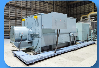
Rewinding Stator Generator " NISHISHIBA " 43,750 kVA. 11,000 V. 2,297 A. 1,500 RPM.
